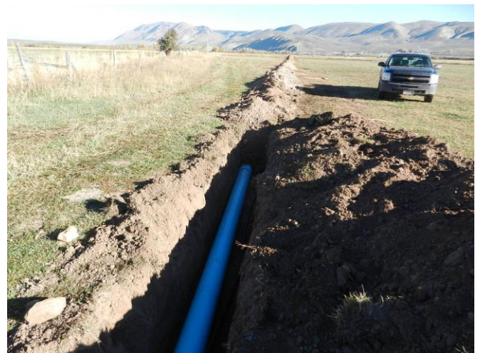
A pipeline being installed in south Lincoln County to assist a producer improve water efficiency
